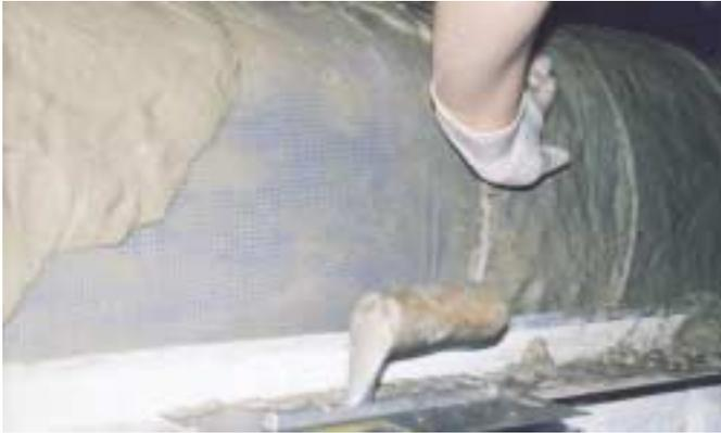
Fig. 4: Hand placement of a 0.2-in. (5.1 mm) thick layer of concrete. Flexible plastic tubing (next to hand) was used to gauge the thickness
